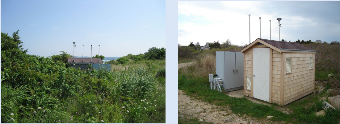
Image 2 Improve site and Air Monitoring Station
